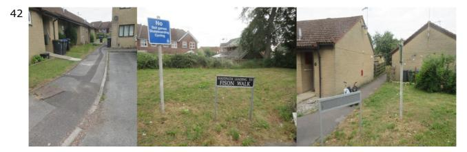
Footway in Hallum Close leading to Fison Walk. Many of the residents of Fison Walk are elderly and less-abled, several appear to use wheelchairs. This drop-kerb and footway are alike in poor condition, and are representative of general conditions.
