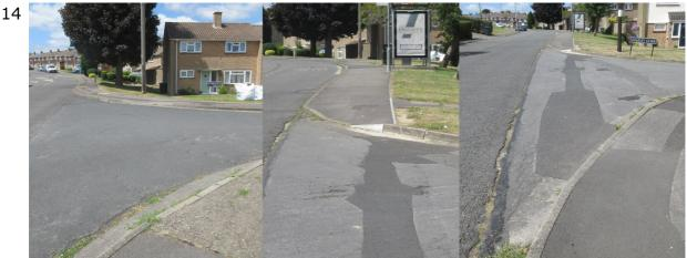
Drop-kerbs. First image is Bingham Road and Bishopdown Road by Catholic Church, very poorly done. Second & Third are upper entry of Hoadley Green, the drop-kerb is only applied to one-third width of the pavement, it stands proud of the road, the surface of which is poor.
