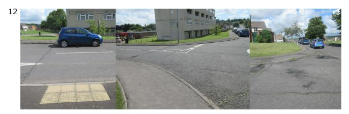
Drop-kerb crossing point of Bishopdown Road by Bishop's Court flats – a car is impeding the crossing point, therefore thought should be given to marking this as a proper crossing point. Similarly, at the junction of Barrington Road with Bishopdown Road there is no crossing point at all for wheelchair and other less able users. Thirdly, the entrance of Gilbert Way has no drop kerb crossing point at all.
