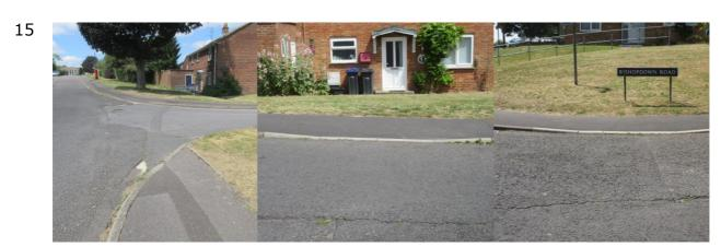
Drop-kerbs. First is lower entry to Hoadley Green, again really poorly done with degraded road surface, proud stones and uneven and narrow paving. Second and Third are drop-kerb crossing point at bottom of Bishopdown Road, the kerb stones again proud.
