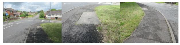
Junction of Bishopdown Road and Denison Rise (right). This steep section of footway is bumpy and degraded, especially where the inspection cover is, part of the inspection cover frame stands clear and is a tripping hazard. This whole section needs relaying.
