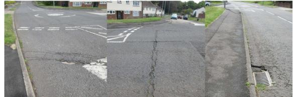
Broken road surfaces above, and below, the roundbout junction of Bishopdown Road and Denison Rise. Below the junction, this drain has sunken hazardously.
