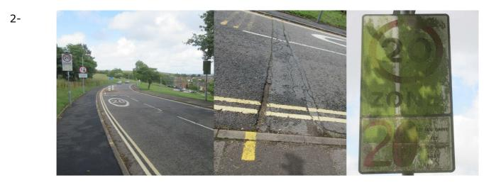
Entry of 20mph zone, top of Bishopdown Hill. The 20mph sign is filthy, mostly due to being close to tree overhang. Adjacent to it a trench in the road needs filling again.
